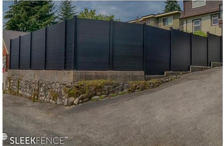
Metal Perimeter Fence
